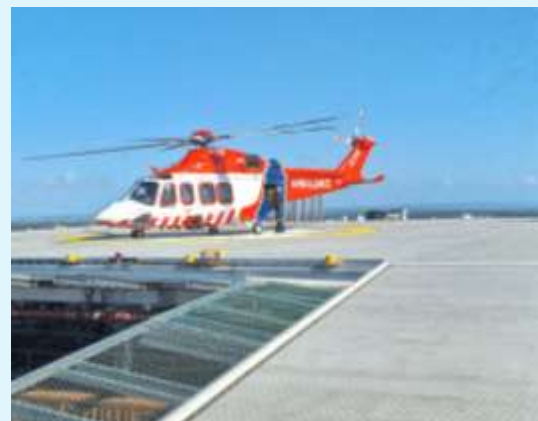
Victorian Heart Hospital - Helipad
